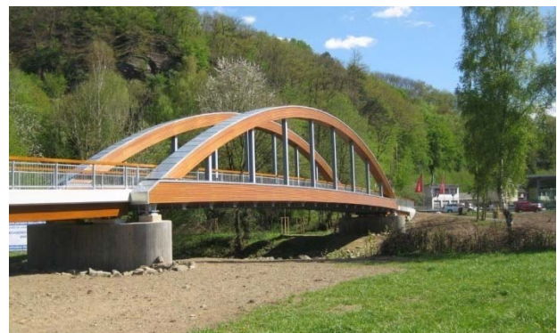
Figure 4: Timber bridge in Hönigesberg (North-Rhine-Westphalia, Germany)
