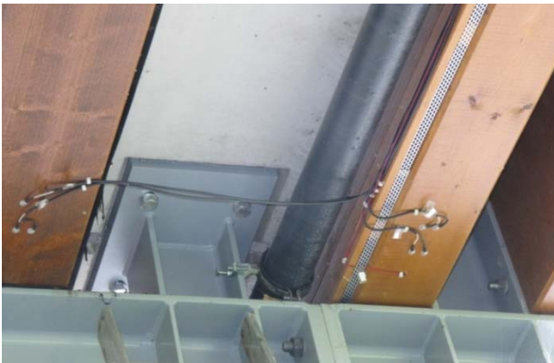
Figure 5: Measuring points of timber moisture and timber temperature above the river
