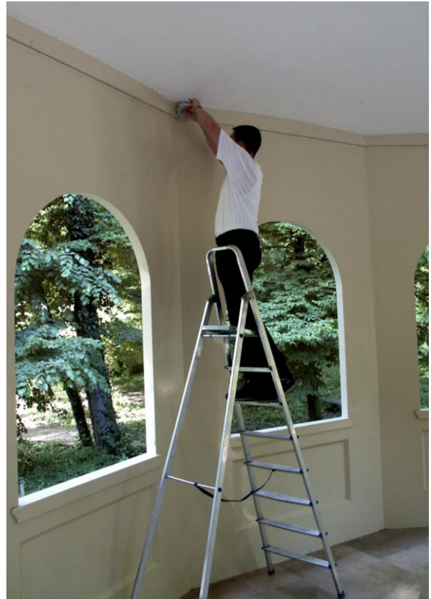
Figure 7: Installation of moisture monitoring device. Left: Position of the three measurement points in the roof. Right: Installation of data logger box.
